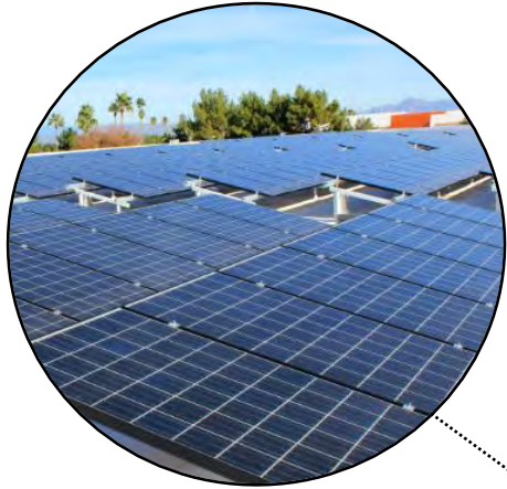
Maximize PV Panels on Roof
