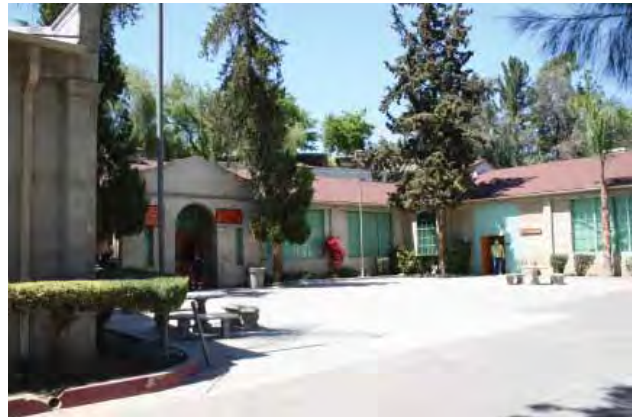
Tehcnology A building in board formed concrete
