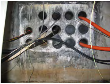
CMH #3 Looking North to CMH #2
