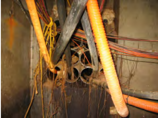
CMH# 02 EAST WALL 1 OF 2
