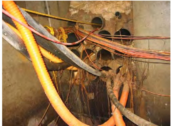
CMH# 02 EAST WALL 2 OF 2
