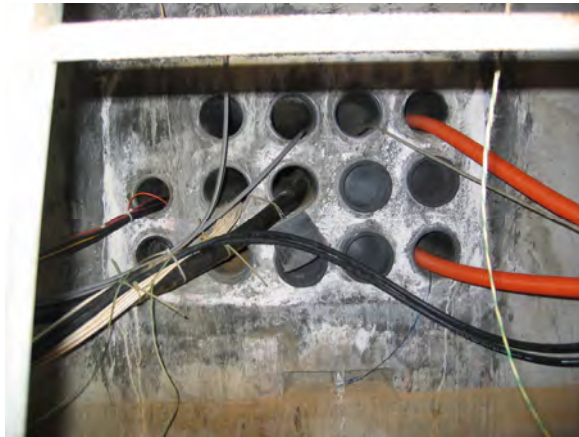
CMH #3 Looking North to CMH #2
