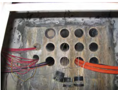
CMH #1 Looking South to CMH #2
