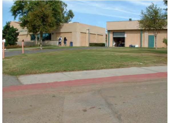
Two 4 inch conduits to Tigers Den
