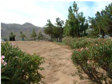
Two 4 inch conduit to HH BB
