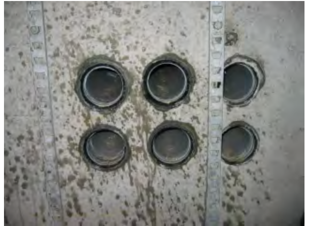
CMH # 03 NORTHWEST WALL
