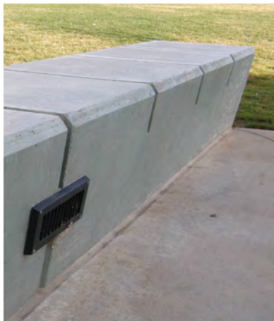
Wall recessed fixture with glare shield
