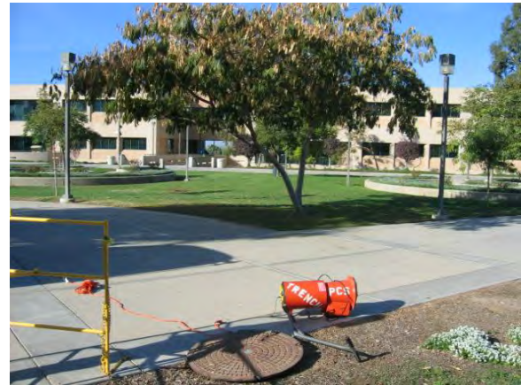
CMH #5 Looking West to CMH #2
