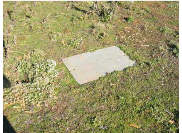
Fire Alarm Pullbox "PB-1"
