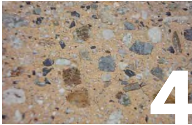
EXPOSED AGGREGATE CONCRETE
