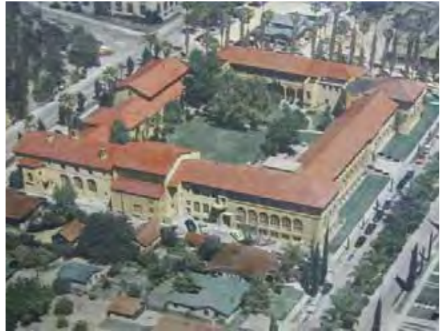
AG Paul Quadrangle building in the California Mission Revival style
