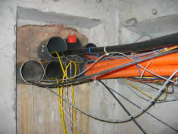
CMH#01 SOUTHWEST WALL
