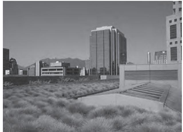
Vancouver Public Library's green roof application
