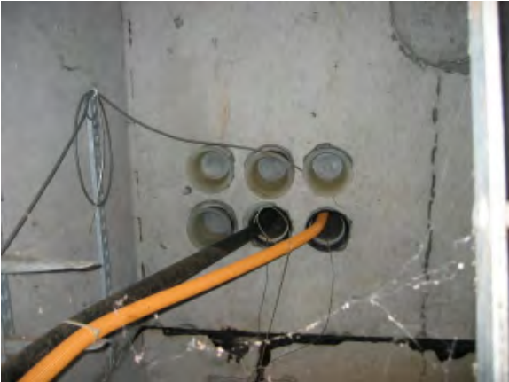
CMH # 04 SOUTHEAST WALL
