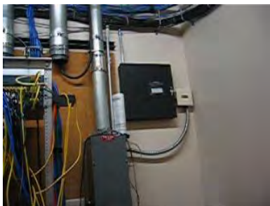
Typical Building Fire Alarm Module
