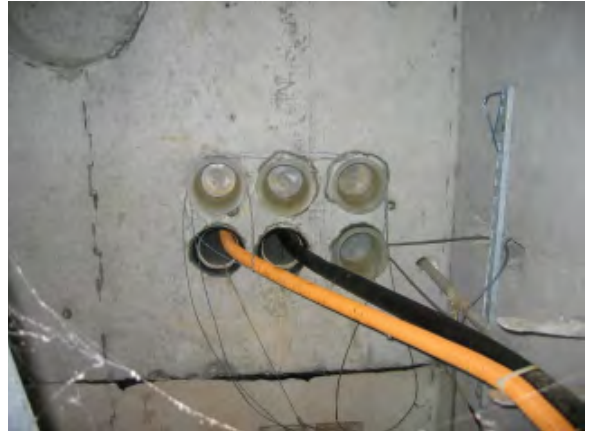
CMH# 04 NORTHEAST WALL
