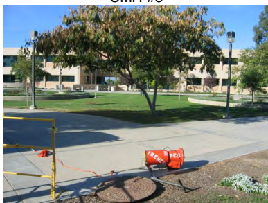
CMH #5 Looking West to CMH #2
