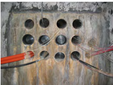
CMH #1 Looking North to Mech-1 Bldg
