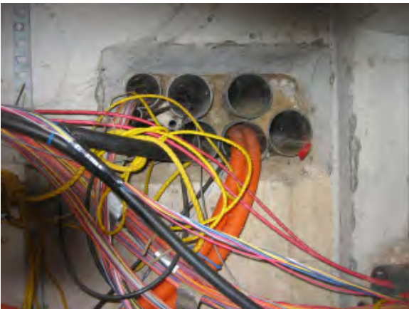
CMH # 01 NORTHEAST WALL
