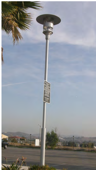
Ellipsoidal post top fixture with full cutoff
