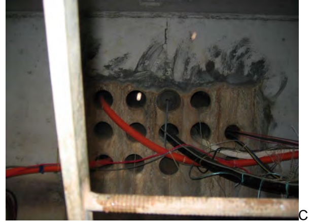
MH #2 Looking South to CMH #3
