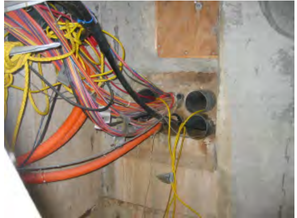
CMH# 01 NORTH EAST WALL
