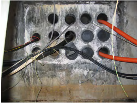
CMH #3 Looking North to CMH #2
