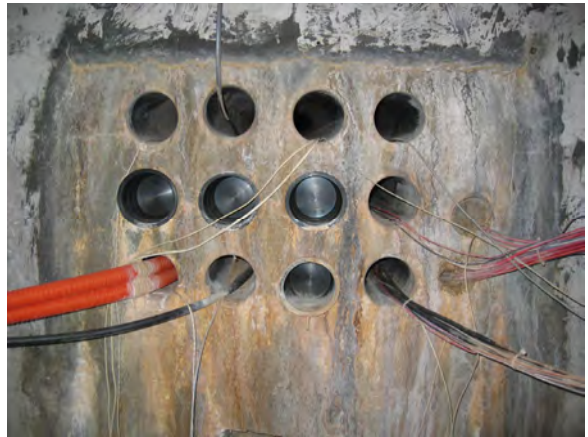
CMH #1 Looking North to Mech-1 Bldg
