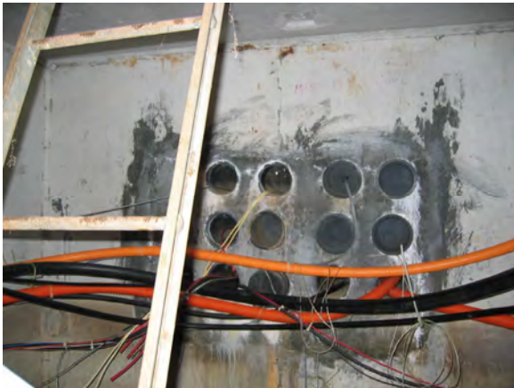
CMH #2 Looking North to CMH #1
