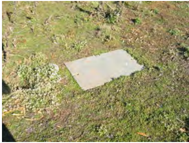
Fire Alarm Pullbox "PB-1"
