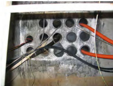
CMH #3 Looking North to CMH #2
