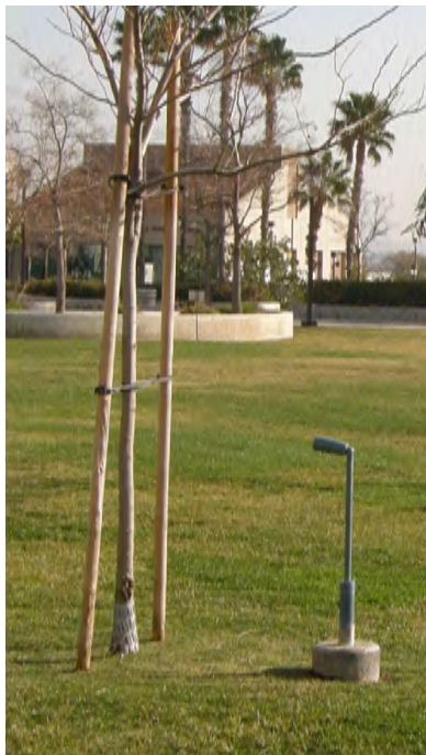
Tree Accent light mounted on 2 foot stake + concrete base painted green
