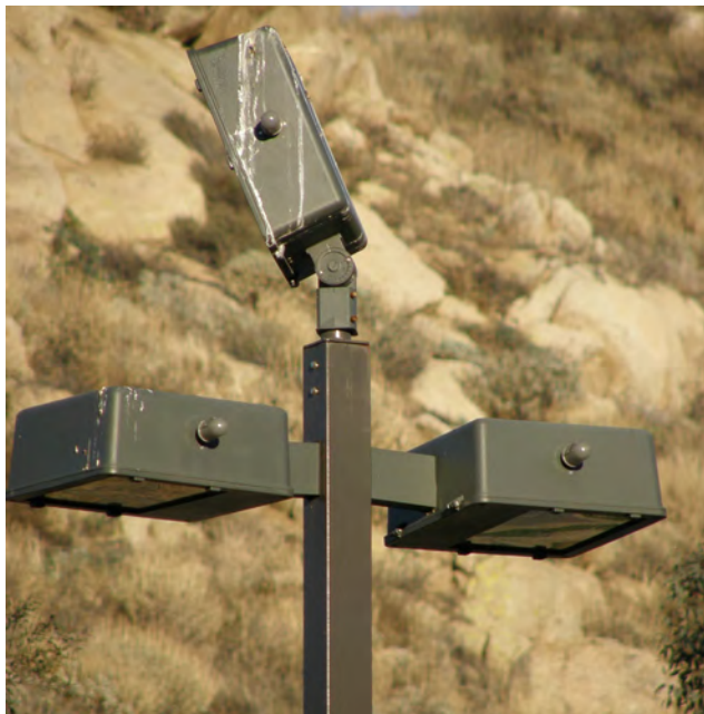
Shoe Box Fixtures-1-3 Heads: MH lamp
