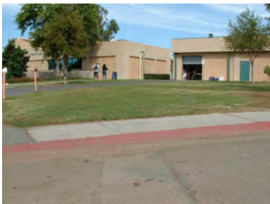
Two 4 inch conduits to Tigers Den
