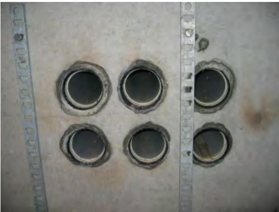
CMH # 04 NORTHWEST WALL
