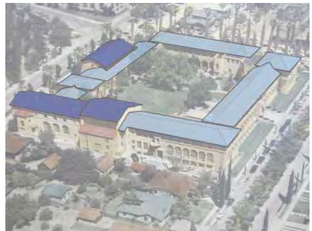
Quadrangle Diagram - Hip and Gabled roofs
