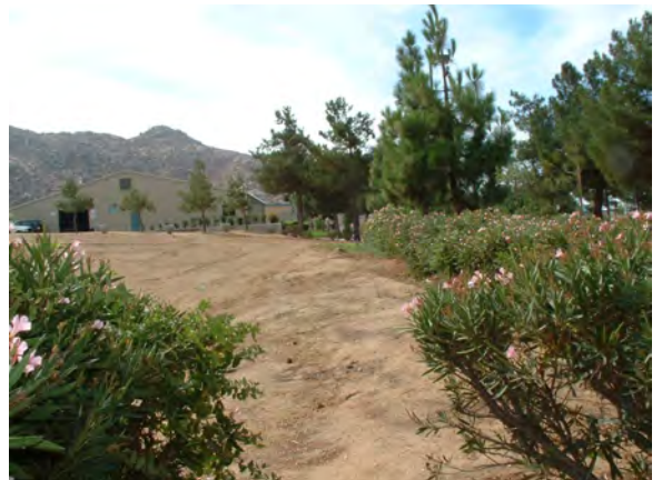
Two 4 inch conduit to HH BB
