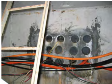
CMH #2 Looking North to CMH #1
