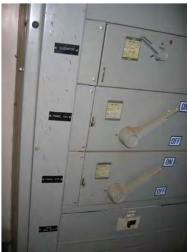
Multipurpose Bldg DPA
