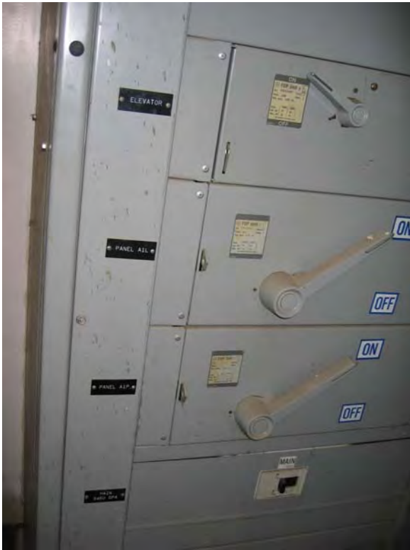
Multipurpose Bldg DPA
