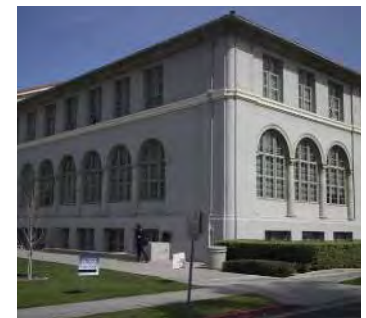
4. Corner of Quadrangle Building ●
