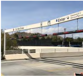
5. Parking Structure Entrance
