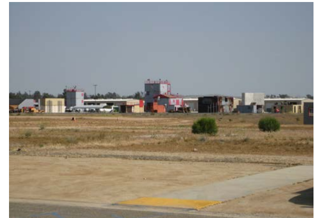
2014 view of BCTC Live-Fire Fire Technology Training Area
