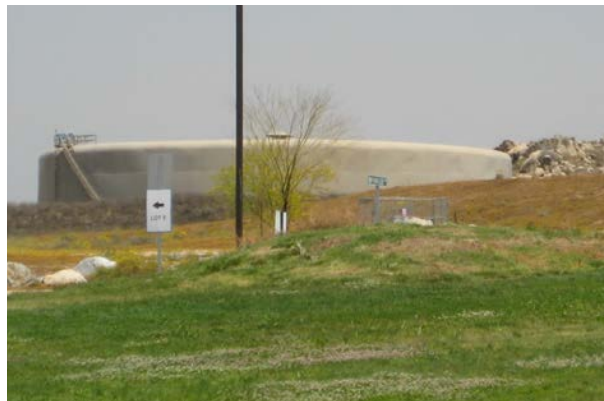
EMWD Water Tanks
