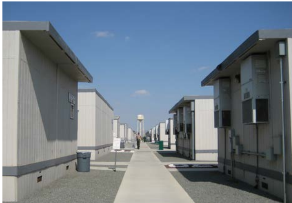
Law Enforcement temporary relocatable classrooms
