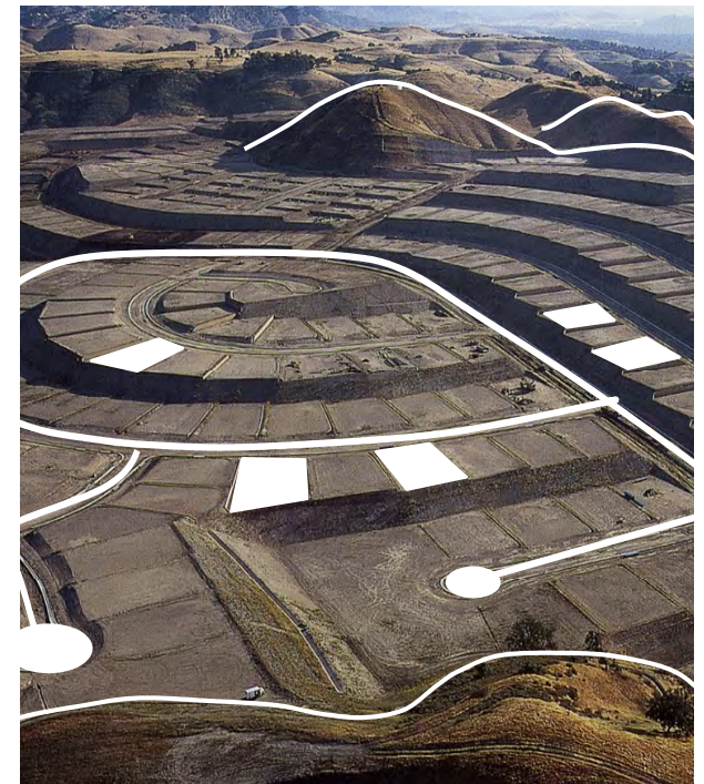
Site preparation for new hillside housing development
