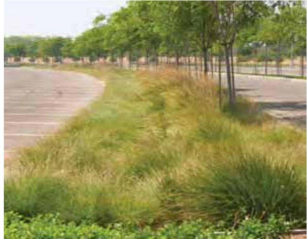
parking lot swale, Veritas Campus II / Milpitas, California
