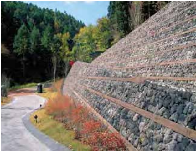
Gabion Wall, Kunming Eco Community/ Kunming, China
