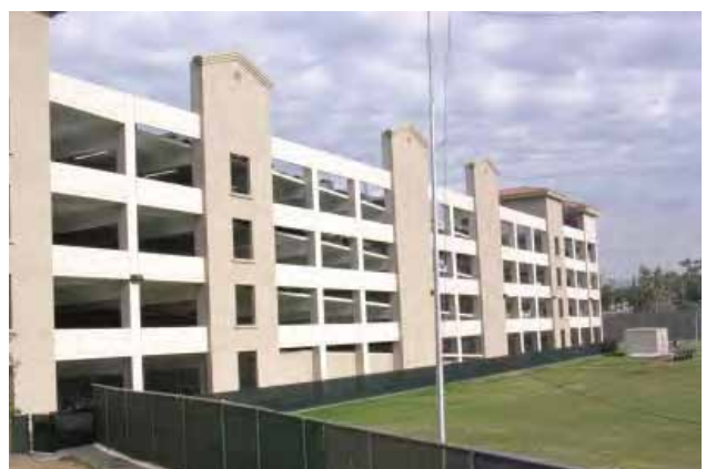
New parking structure on campus
