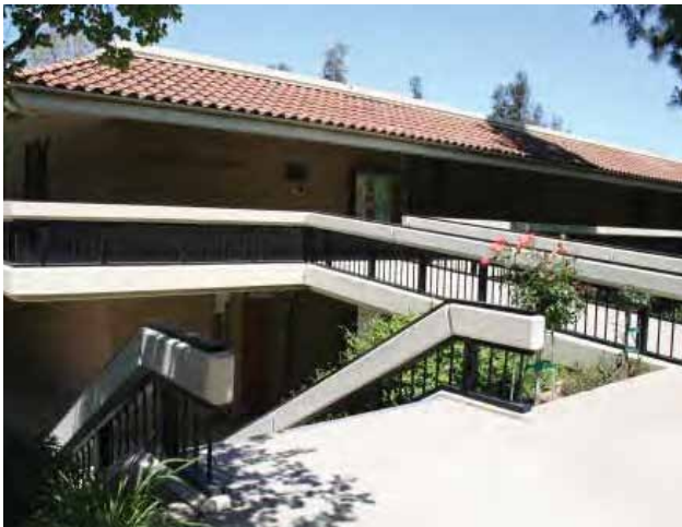
Site topography requires a variety of building approaches to negotiate grade changes
