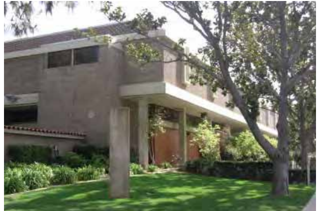
Martin Luther King, Jr. Library with concrete block
