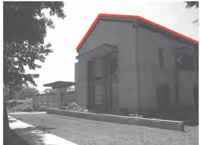
Gabled roof at Claremont College
