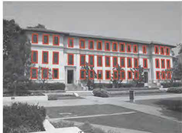
Punched articulation of openings at Occidental College
