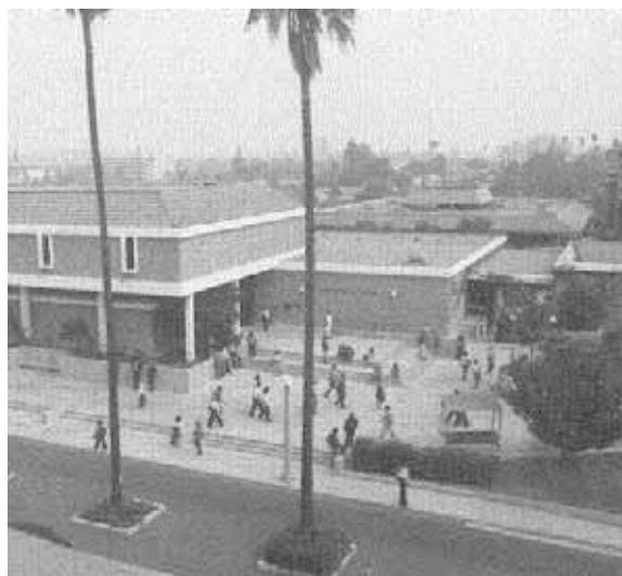
Martin Luther King, Jr. High Technology Center, 1977
