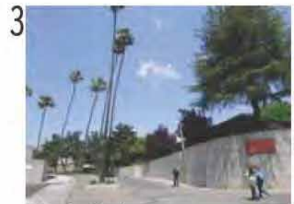
Sloped pedestrian entrance
