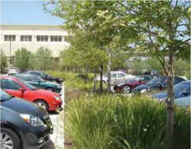
Parking swales, California Endowment / Los Angeles, California
