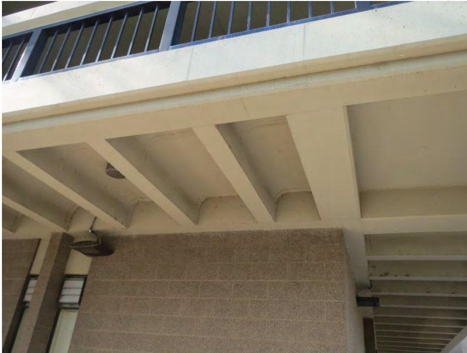
Figure 8. Life Science, Detail, coffered ceiling under cantilevered walkway (IMG_4545)
