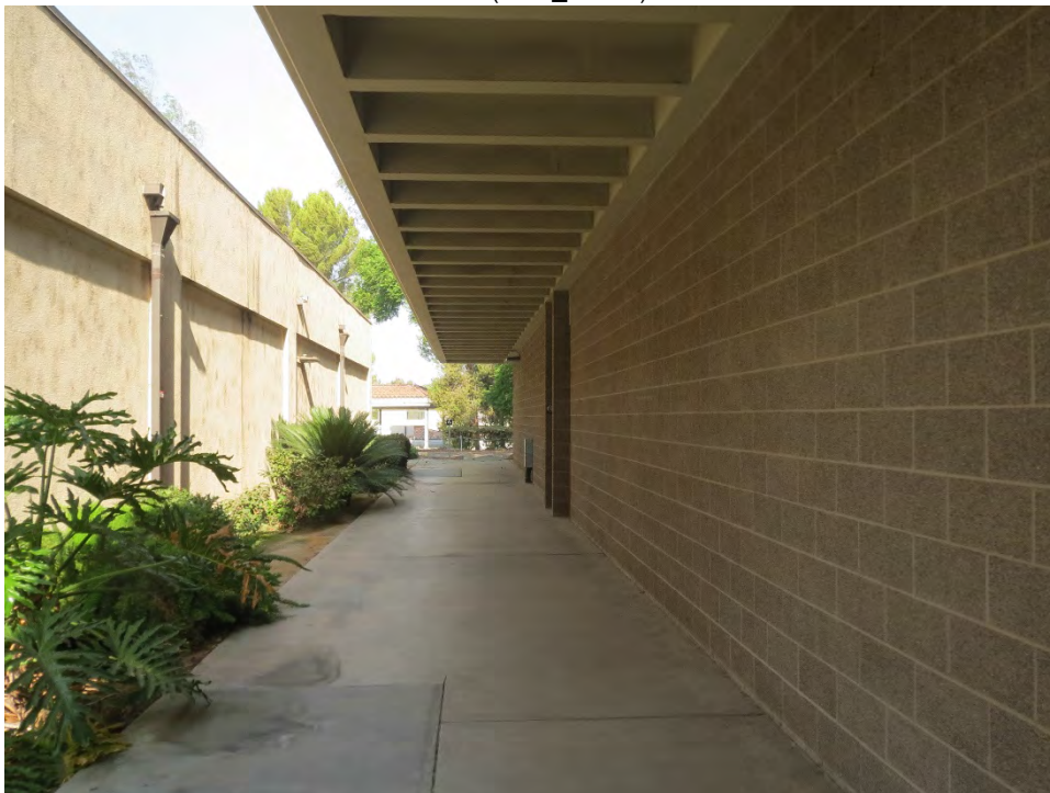
Figure 34. Physical Science Building, first floor of South elevation, looking west (IMG_4503)
