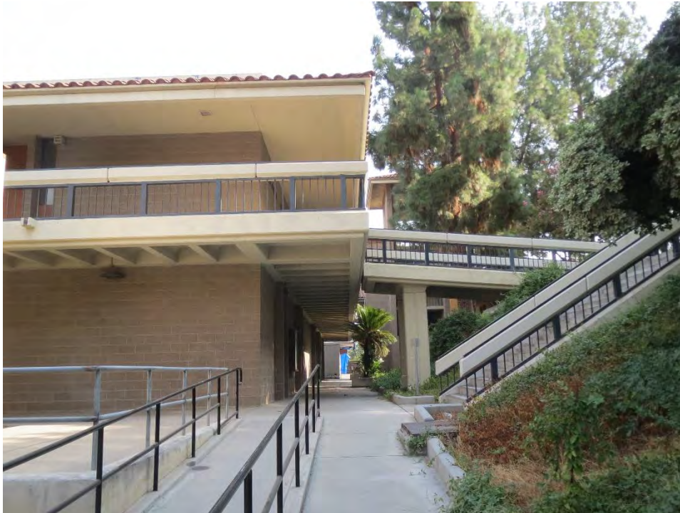
Figure 2. Physical Science Building, portion of South elevation, detail of ramp and stair looking north (IMG 4500)
