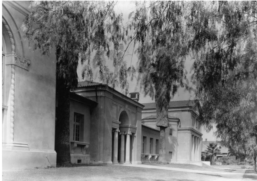
Figure 7. North elevation of the Quadrangle building, facing Terracina Drive (Library, Auditorium, and Memorial Entrance), circa 1932. (Security Pacific National Bank Collection, Los Angeles Public Library)
