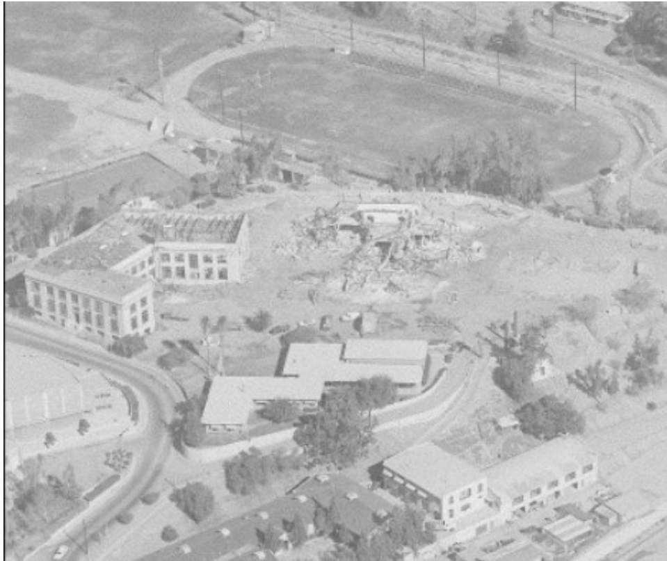
Figure 11. Demolition of the Polytechnic High School buildings, 1965. (Steinberg Architects 2008)
