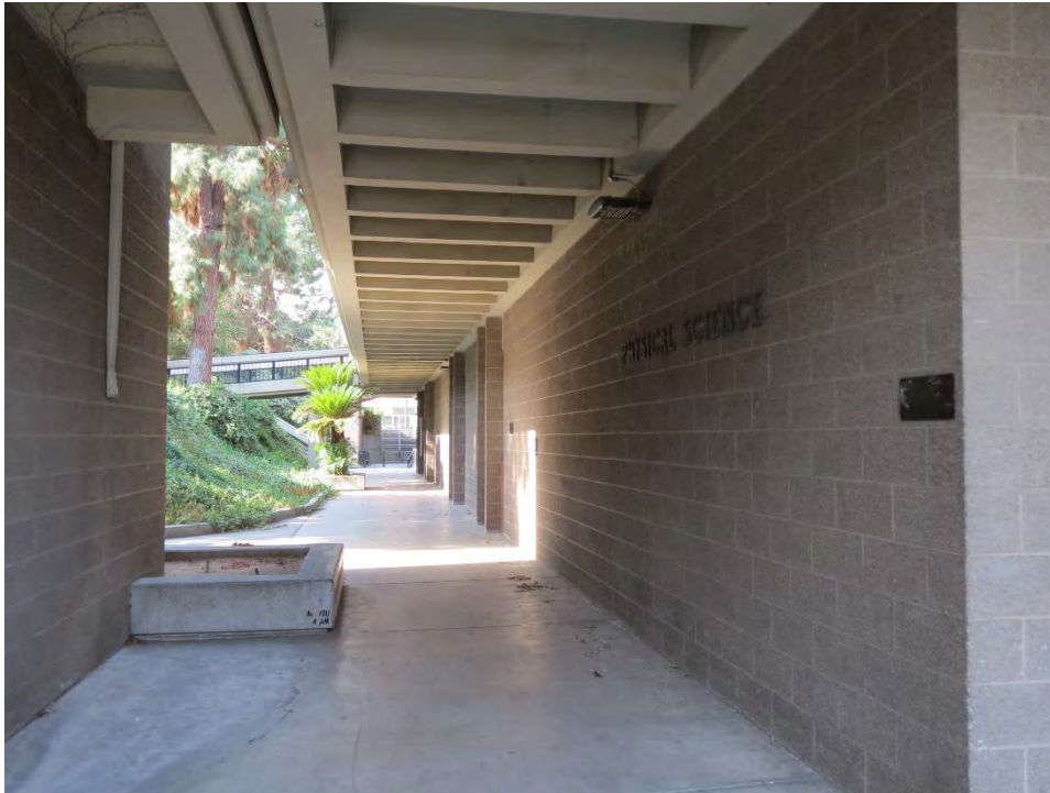
Figure 8. Physical Science Building, East Elevation lower level walkway, looking south (IMG_4564)
