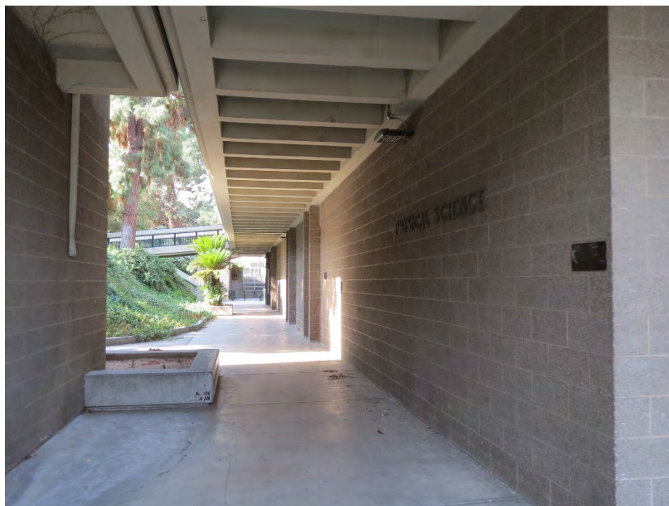
Figure 39. Physical Science Building, East Elevation lower level walkway, looking south (IMG_4564)
