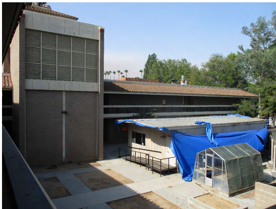
Figure 37. Physical Science Building, North elevation with clocktower at left, portables in front, looking southwest (IMG_5251)
