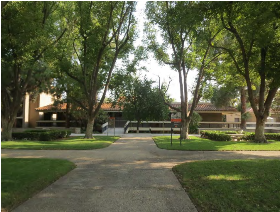
Figure 1. Life Science, Main (south) elevation, looking north (IMG_4487)
