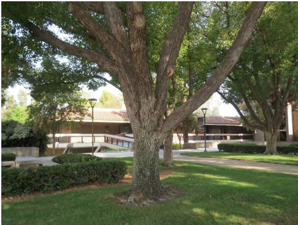
Figure 1. Physical Science Building, main (east) elevation, looking northwest (IMG_4488)
