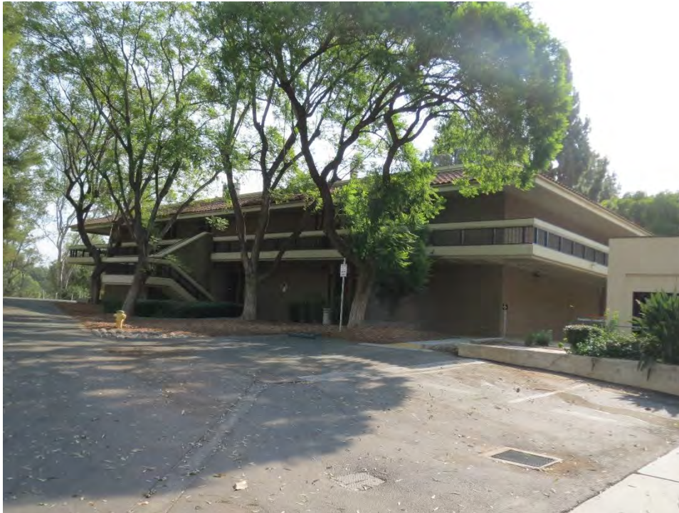
Figure 4. Physical Science Building, South and West elevation, looking northeast (IMG_4509)
