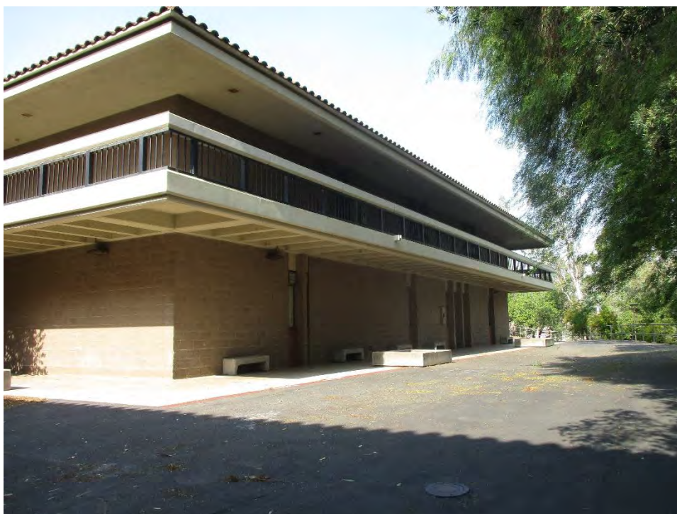
Figure 5. Life Science, North Elevation, looking southwest (IMG_5208)
