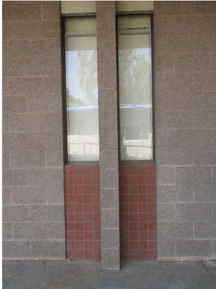
Figure 27. Life Science Building, Detail, paired window (IMG_5221)
