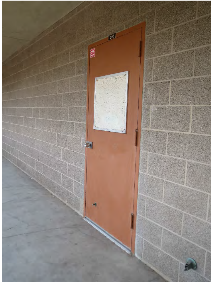
Figure 44. Physical Science Building, detail, atypical door flush with wall (IMG_4590)
