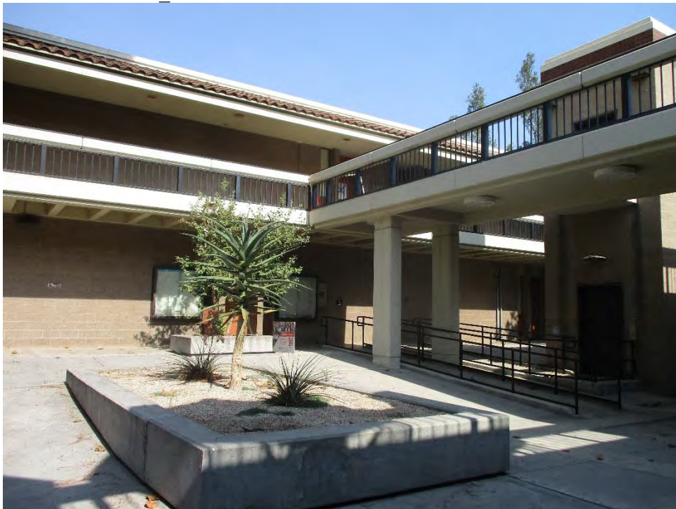
Figure 7. Life Science, portion of east elevation and cafeteria elevated walkway, looking northwest (IMG_5190)
