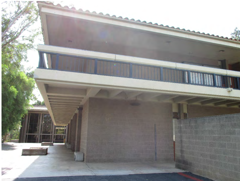
Figure 19. Life Science, portion of West elevation, looking east (IMG_5218)
