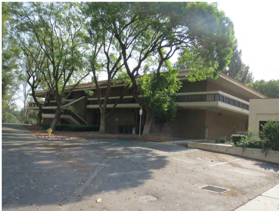
Figure 35. Physical Science Building, South and West elevation, looking northeast (IMG_4509)
