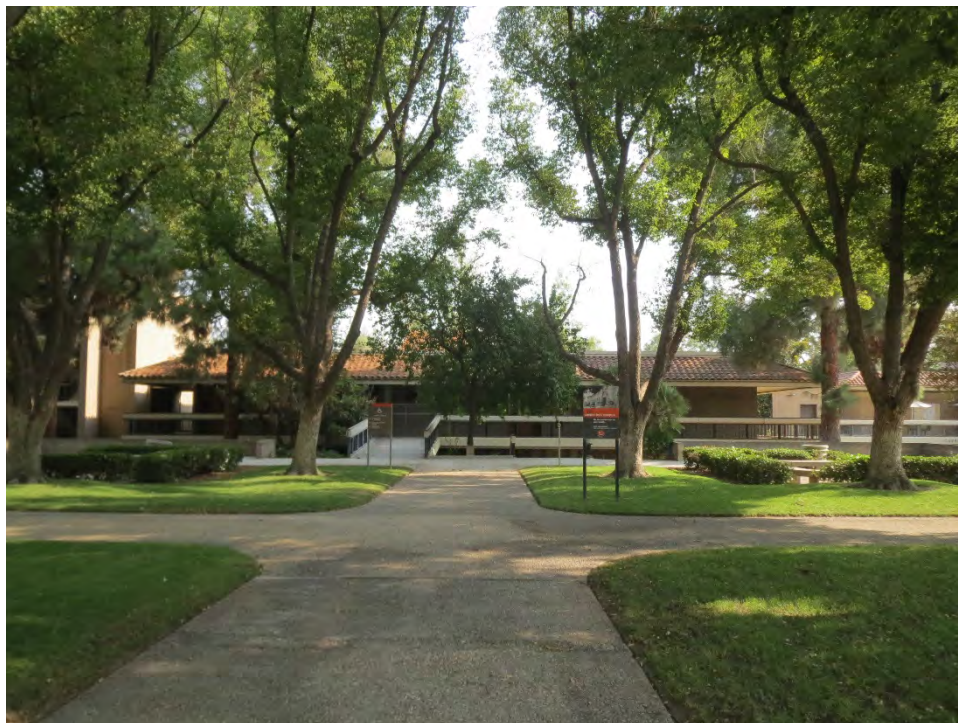
Figure 16. Life Science, Main (south) elevation, looking north (IMG_4487)
