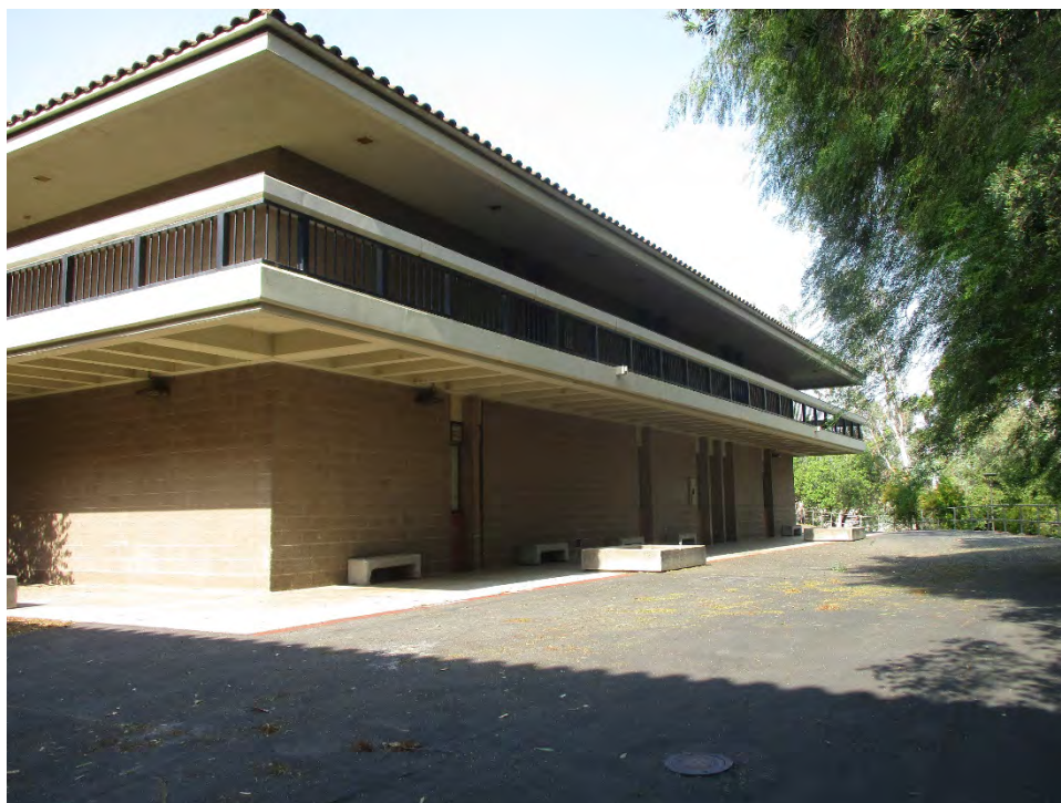
Figure 20. Life Science, North Elevation, looking southwest (IMG_5208)
