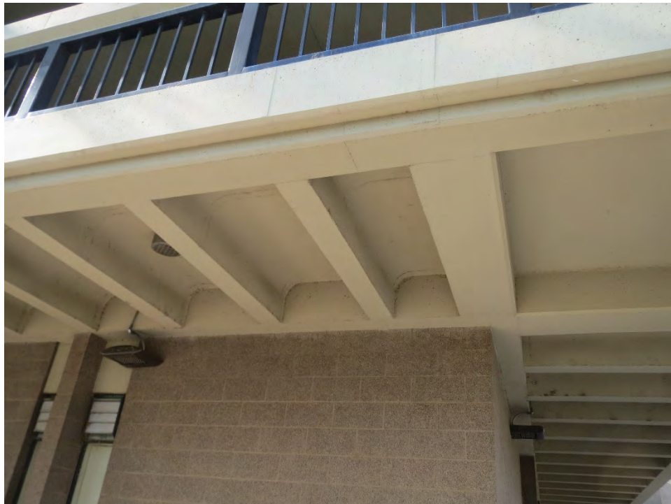
Figure 23. Life Science, Detail, coffered ceiling under cantilevered walkway (IMG_4545)
