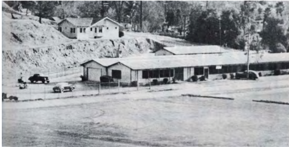
Figure 9. Shop building on Saunders Street, completed 1947. (RCCD 1989)
