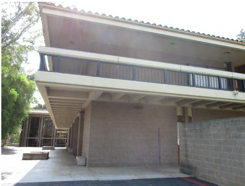
Figure 4. Life Science, portion of West elevation, looking east (IMG_5218)
