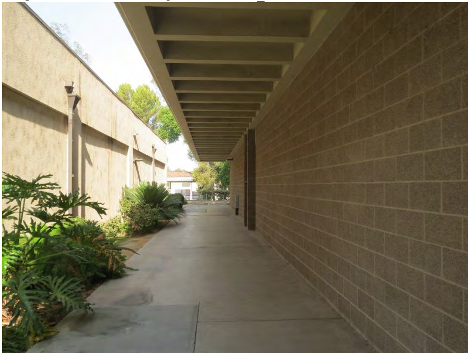
Figure 3. Physical Science Building, first floor of South elevation, looking west (IMG_4503)
