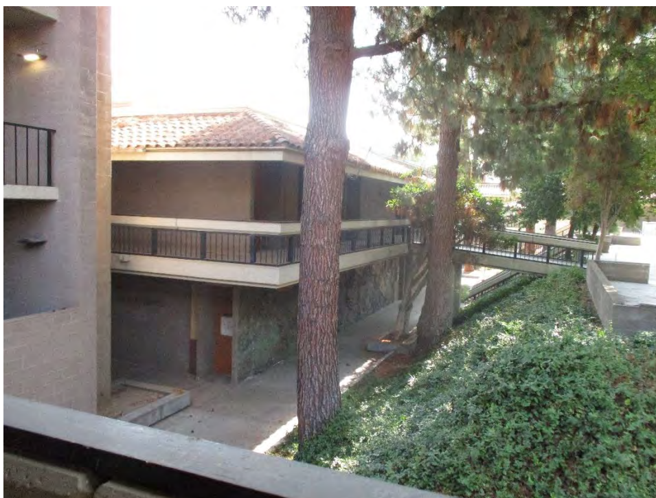
Figure 3. Life Science, portion of West elevation, looking east (IMG_5240)
