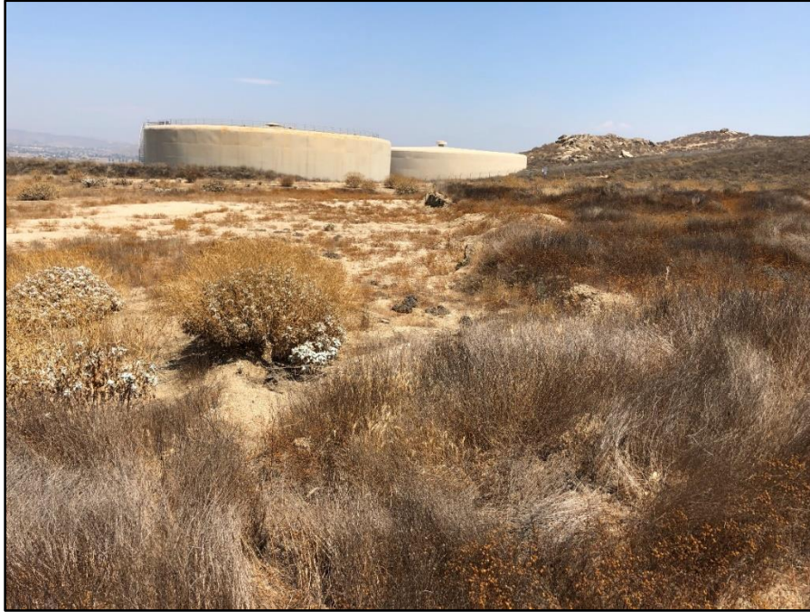
Image 11. View of PV Solar Array Work Area, looking northeast (IMG_2095)
