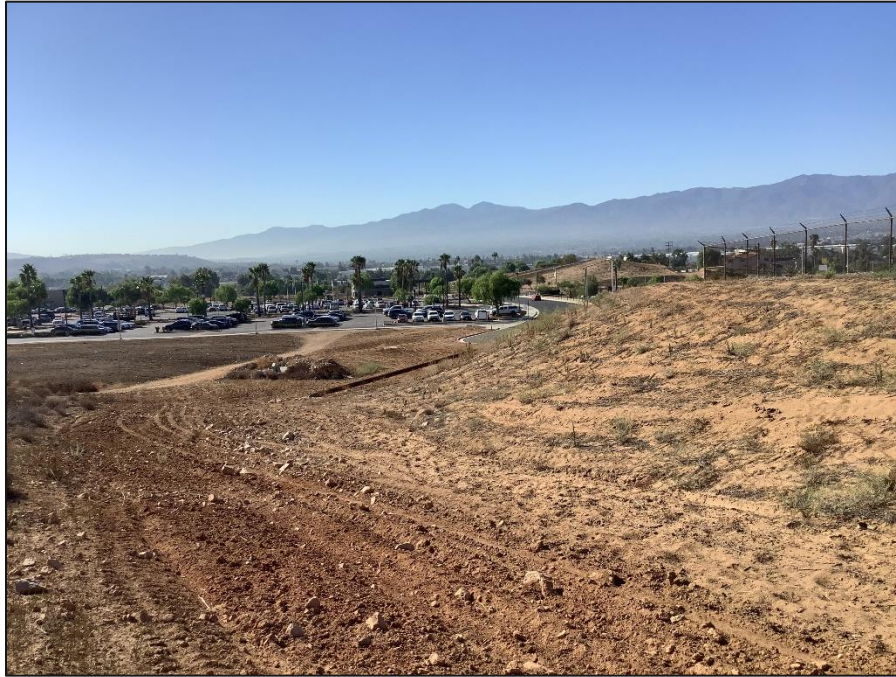
Image 9. View of area where route of New 12 kV Underground line would exit the vacant/undeveloped area towards the campus, looking south/southwest (IMG_0679)
