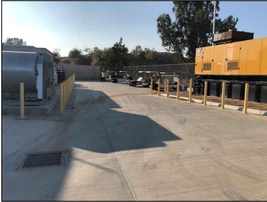
Image 1. View of BESS Work Area, looking northwest (IMG_2275)
