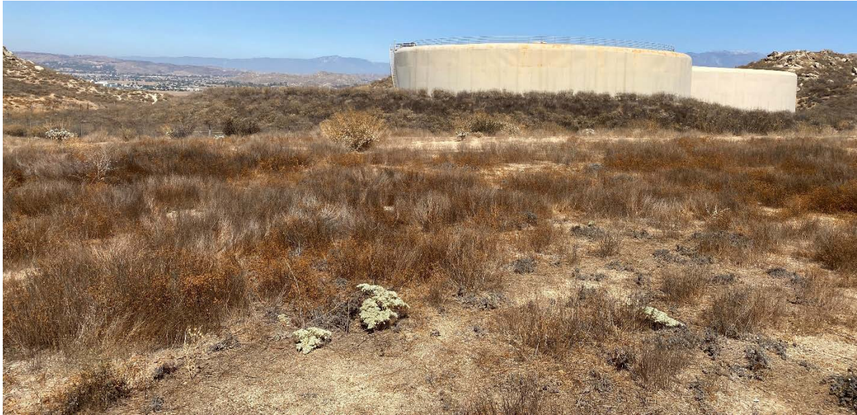
Photograph No. 2: Present proposed site conditions, facing north towards existing reservoirs.
