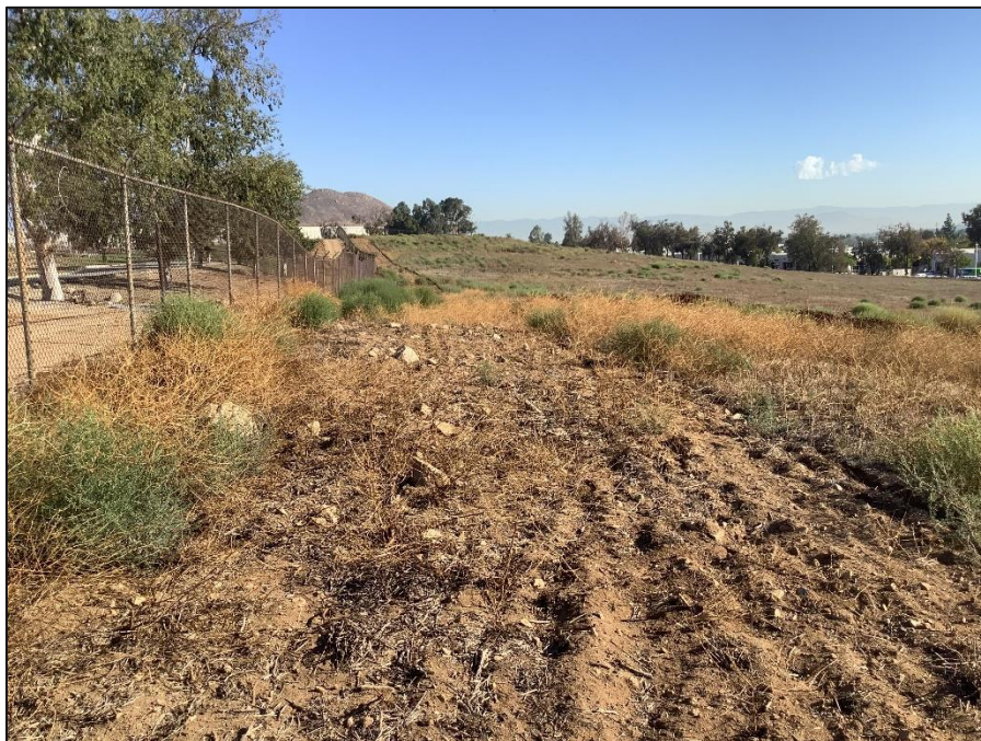
Image 4. View of New 12 kV Underground Line Work Area, looking north (IMG_0657)
