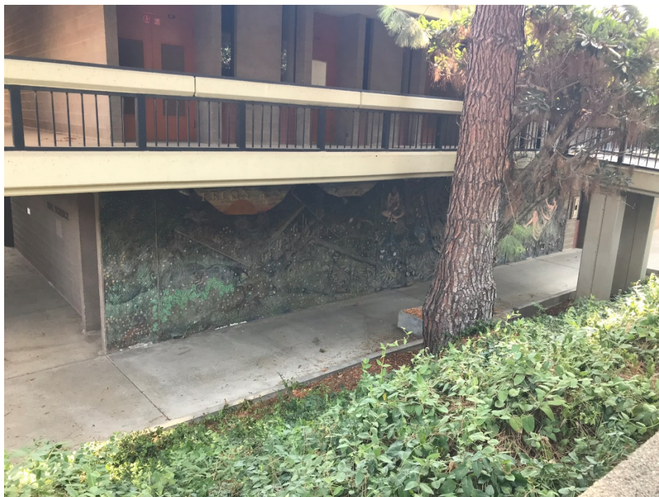
Figure 28. Detail, mural location on south elevation of Life Science Building (IMG_2157)
