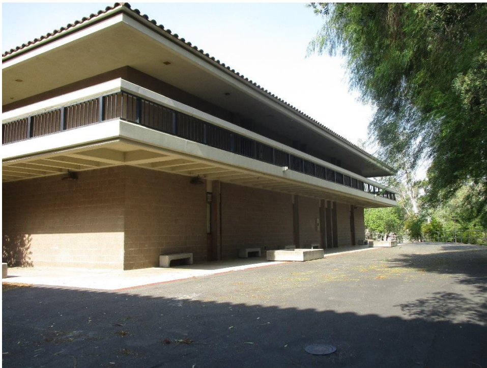
Figure 5. Life Science, North Elevation, looking southwest (IMG_5208)
