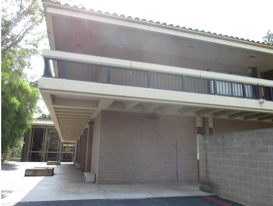
Figure 4. Life Science, portion of West elevation, looking east (IMG_5218)
