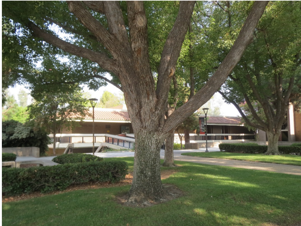
Figure 32. Physical Science Building, main (east) elevation, looking northwest (IMG_4488)
