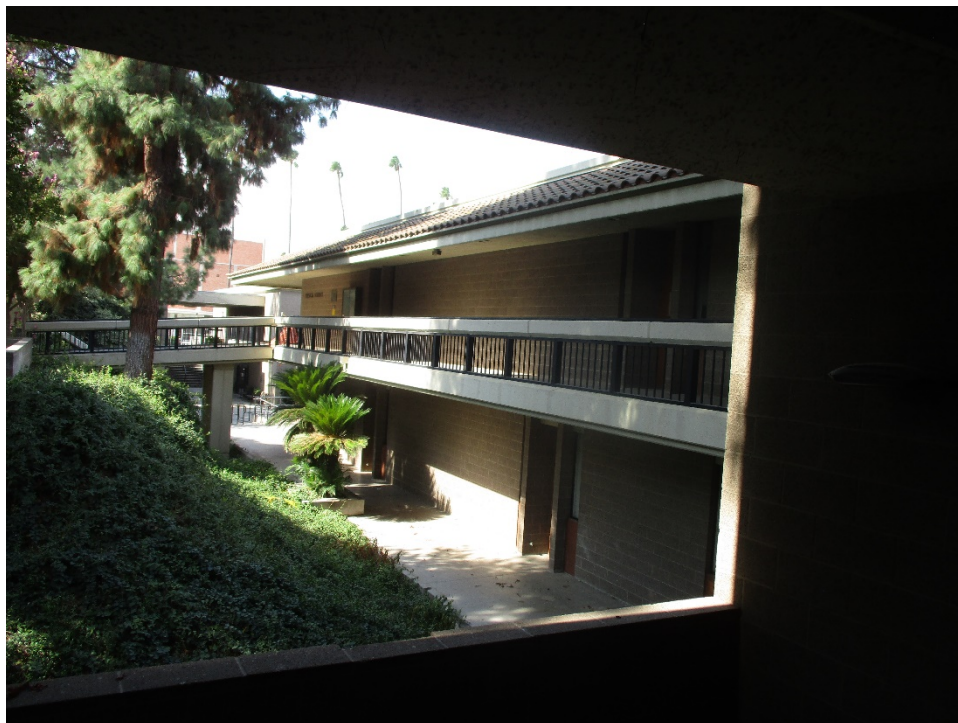
Figure 41. Physical Science Building, East elevation, looking southwest (IMG_5262)
