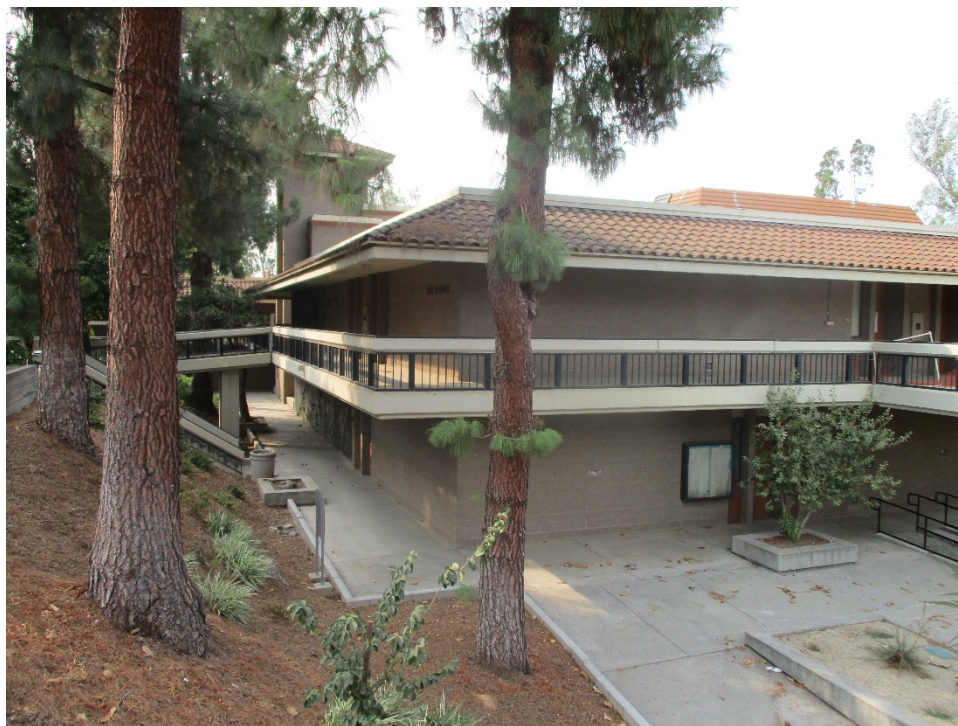
Figure 17. Life Science, East elevation, looking northwest (IMG_5425)
