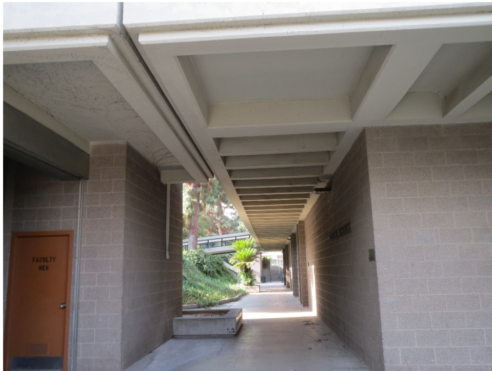
Figure 43. Physical Science Building, detail, coffered ceiling, looking south (IMG_4560)
