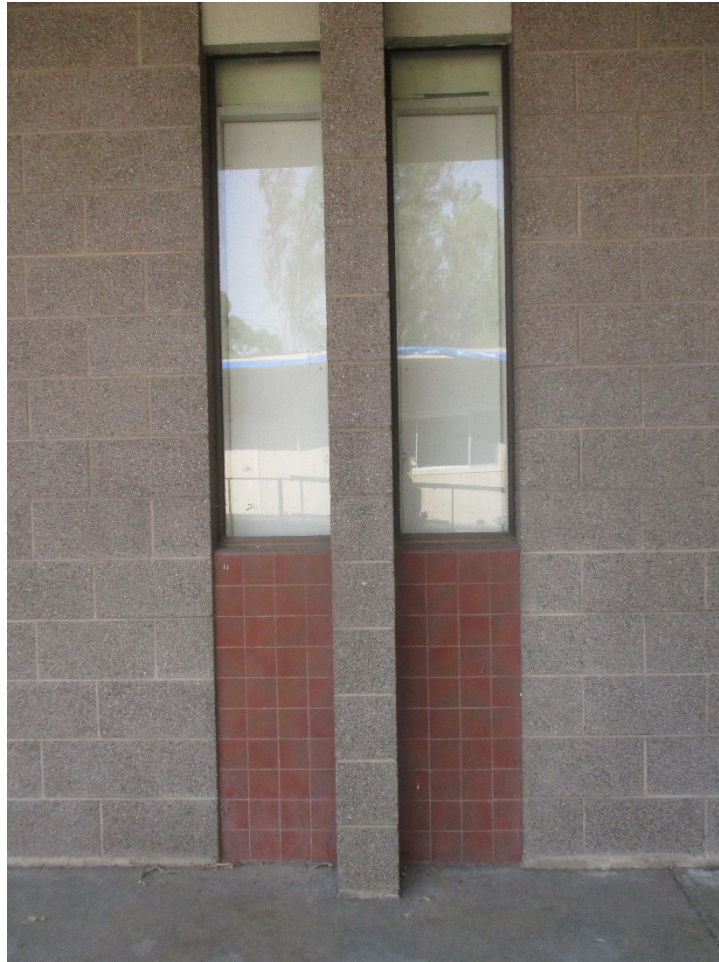
Figure 27. Life Science Building, Detail, paired window (IMG_5221)
