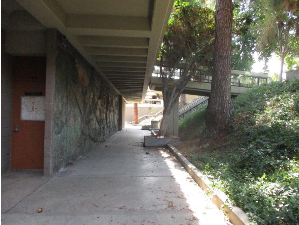
Figure 2. Detail of Mural showing bridge, stair and cantilevered walkway looking east (IMG_5230)
