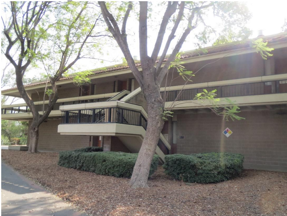
Figure 5. Physical Science Building, detail, stairs on West elevation (IMG_4518)
