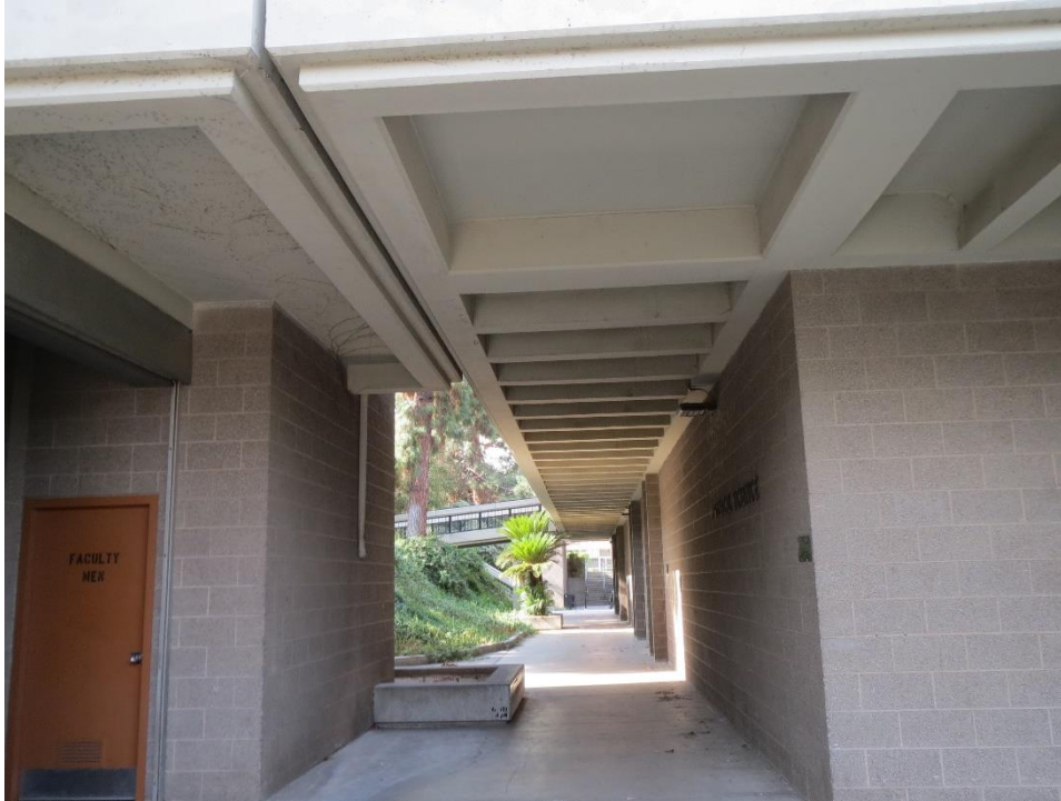
Figure 12. Physical Science Building, detail, coffered ceiling, looking south (IMG_4560)
