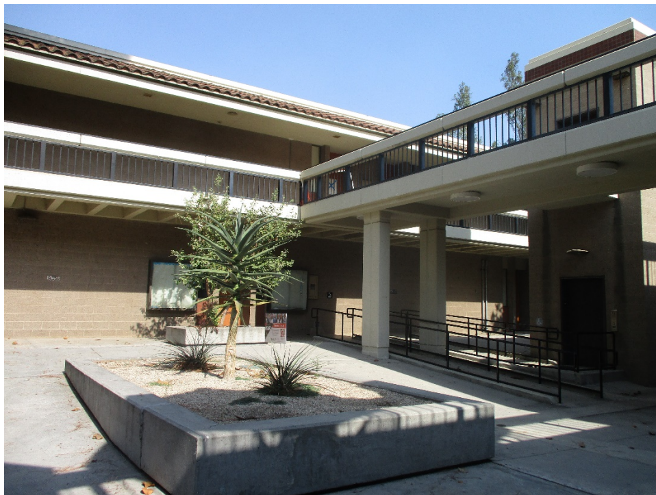
Figure 22. Life Science, portion of east elevation and cafeteria elevated walkway, looking northwest (IMG_5190)
