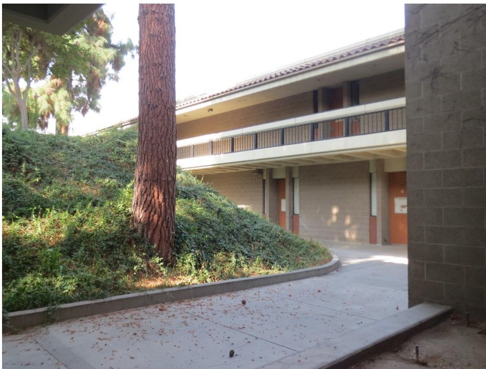
Figure 9. Physical Science Building, East elevation, looking southwest (IMG_4570)
