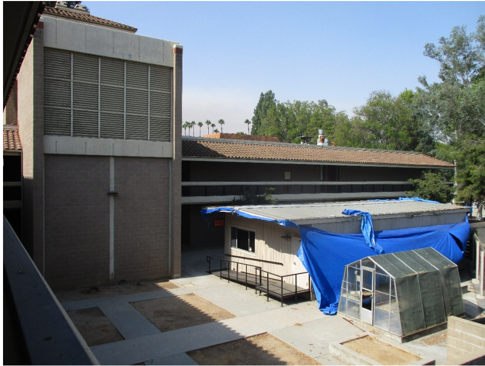
Figure 37. Physical Science Building, North elevation with clocktower at left, portables in front, looking southwest (IMG_5251)
