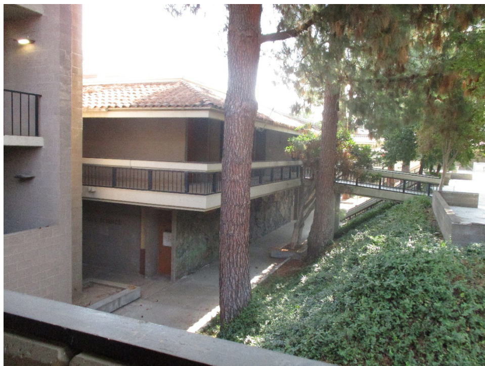
Figure 18. Life Science, portion of West elevation, looking east (IMG_5240)
