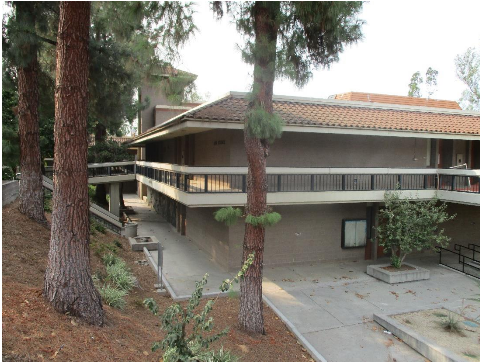
Figure 2. Life Science, East elevation, looking northwest (IMG_5425)
