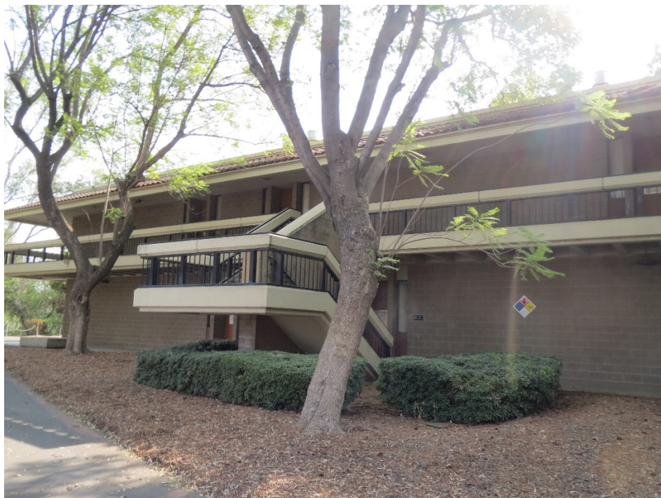
Figure 36. Physical Science Building, detail, stairs on West elevation (IMG_4518)
