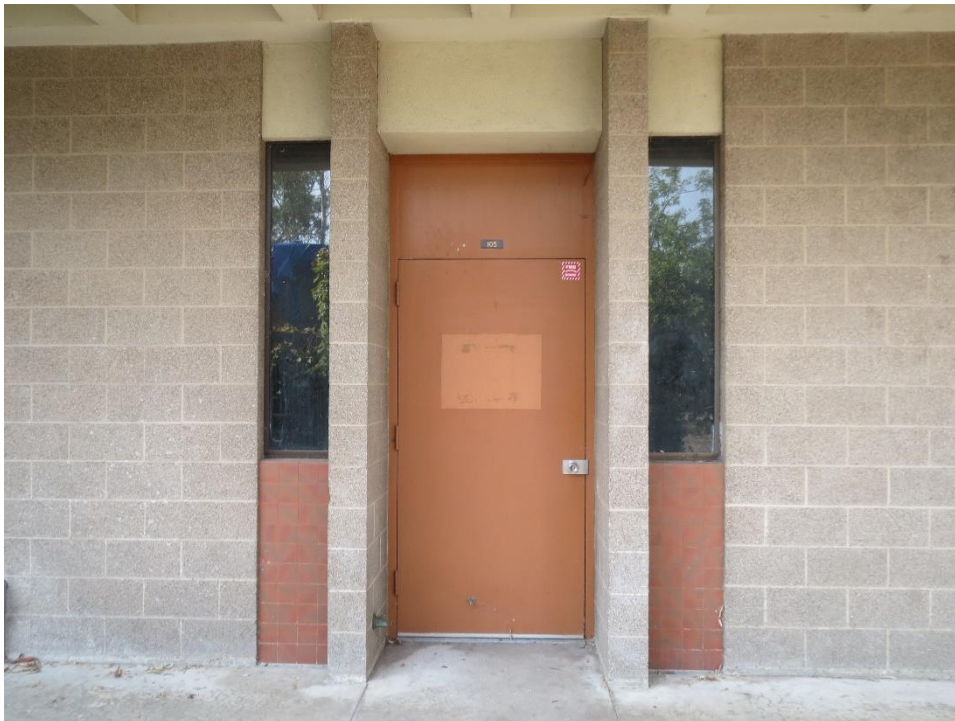
Figure 11. Physical Science Building, detail, typical classroom door (IMG_4532)
