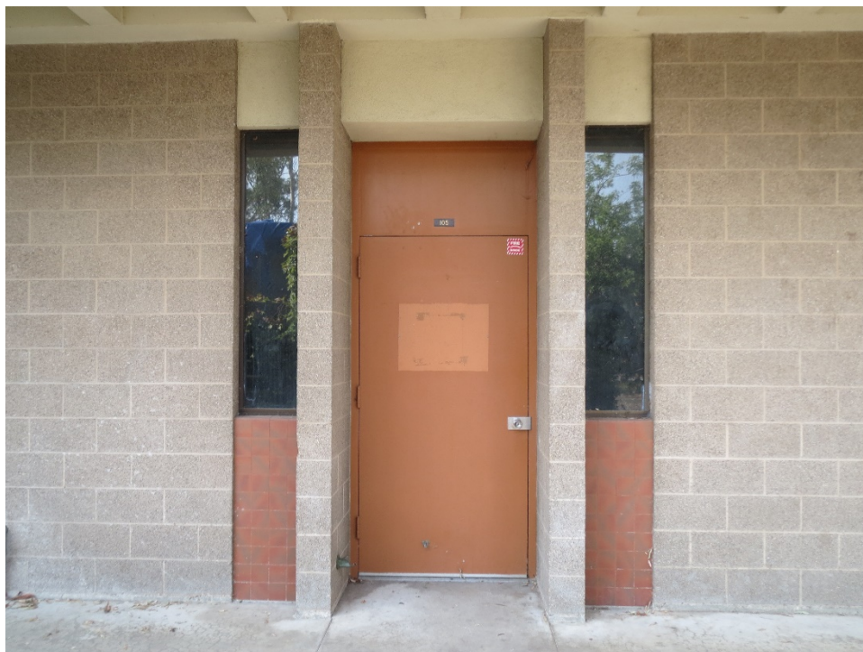
Figure 42. Physical Science Building, detail, typical classroom door (IMG_4532)
