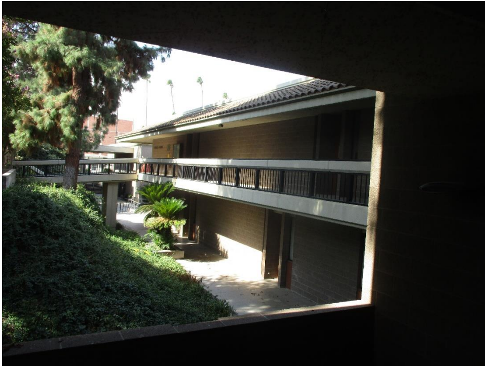
Figure 10. Physical Science Building, East elevation, looking southwest (IMG_5262)
