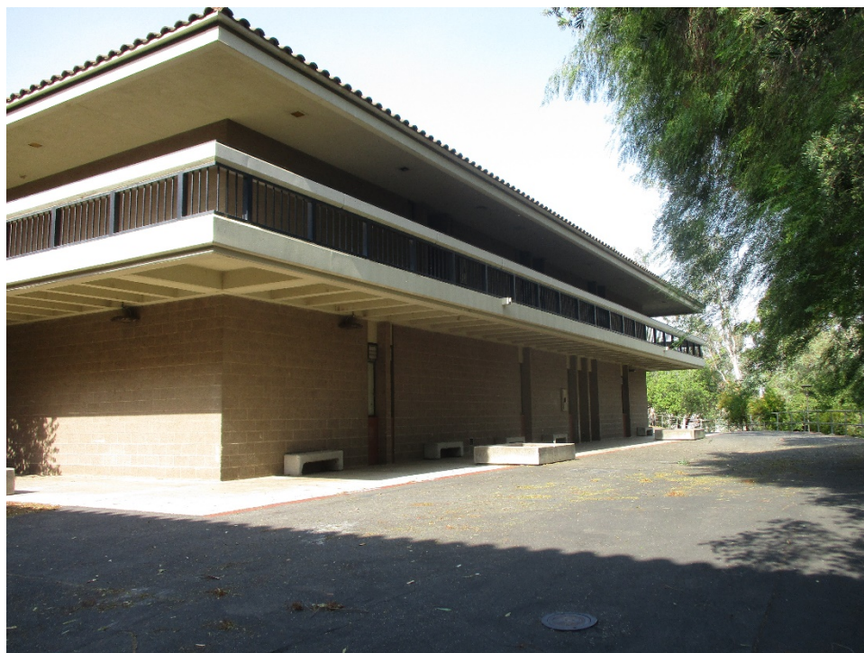
Figure 20. Life Science, North Elevation, looking southwest (IMG_5208)
