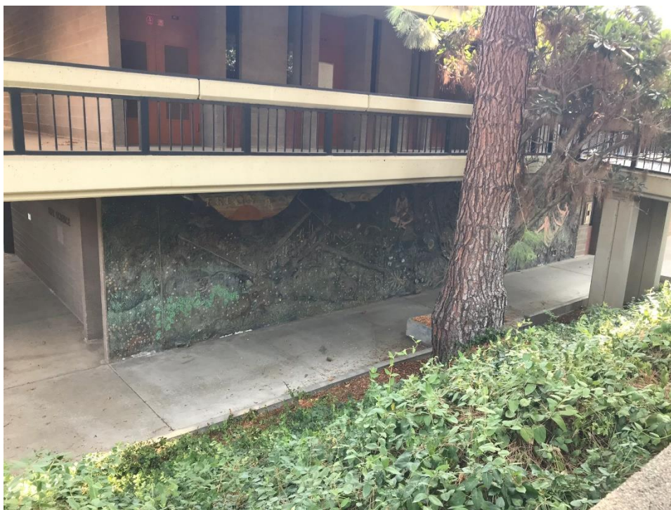
Figure 1. Detail, mural location on south elevation of Life Science Building (IMG_2157)
