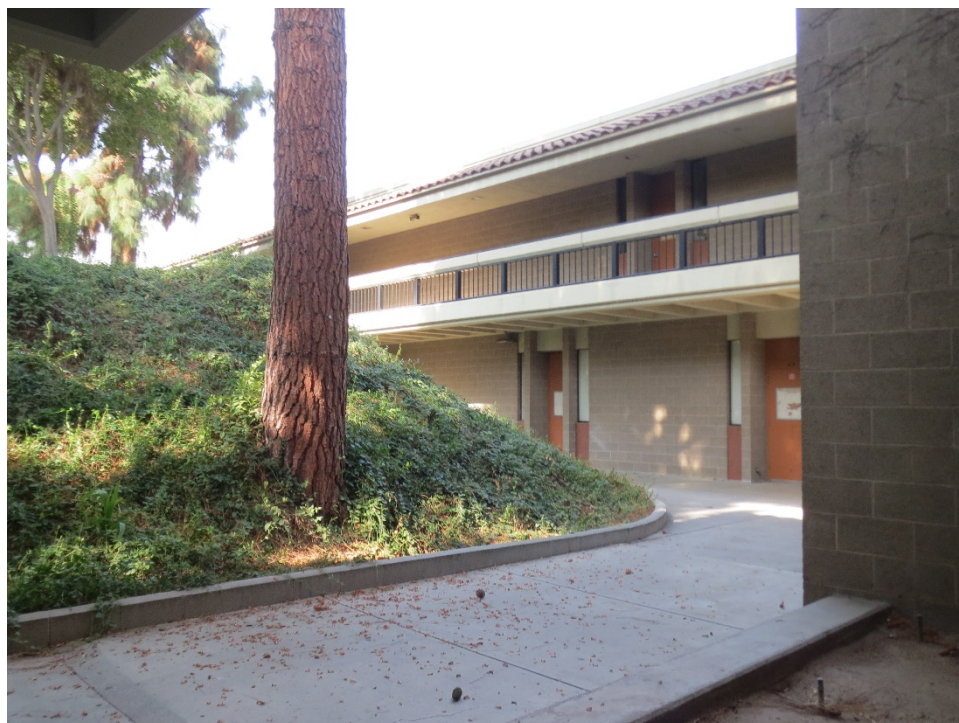
Figure 40. Physical Science Building, East elevation, looking southwest (IMG_4570)
