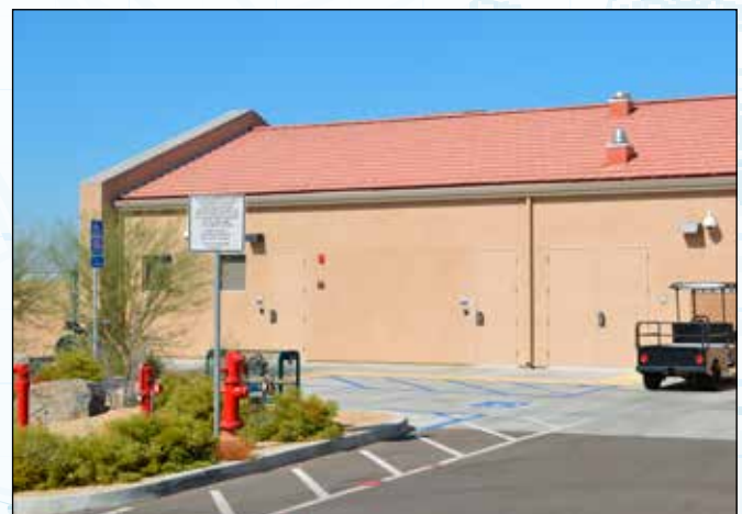
Network Operations Center at Moreno Valley College
