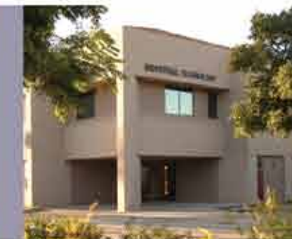
Industrial Tech Building, Norco College
