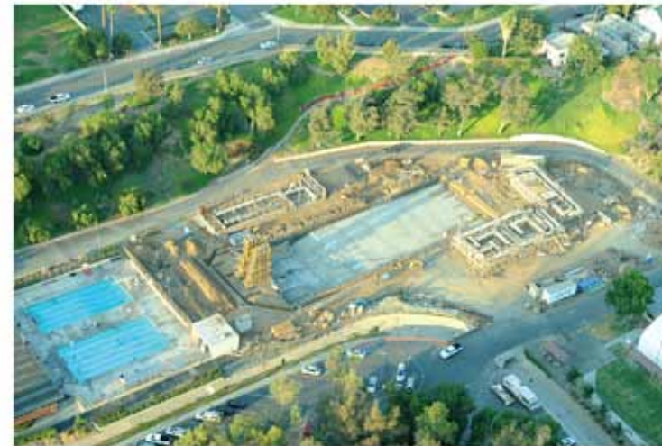
Construction of the Riverside Aquatics Complex, Riverside City College
