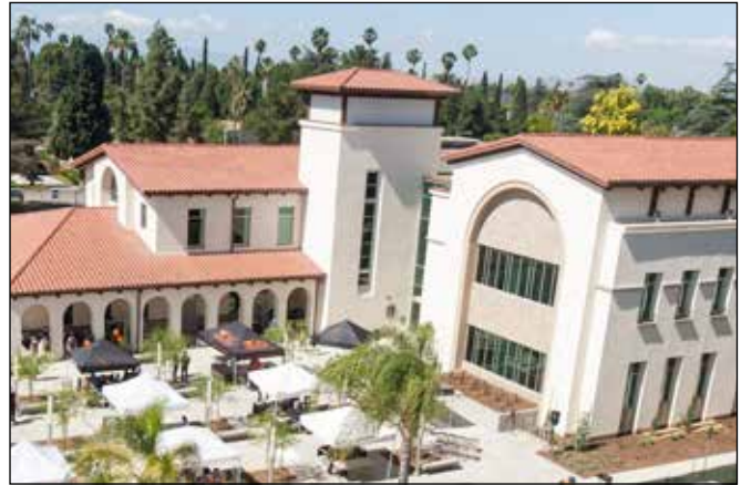
Dr. Charles A. Kane Student Services and Administration Building at Riverside City College
