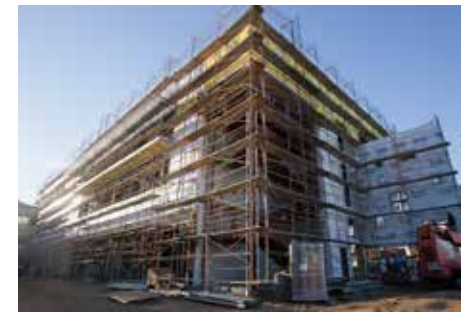
Student Academic Services Building Under Construction, Moreno Valley College
